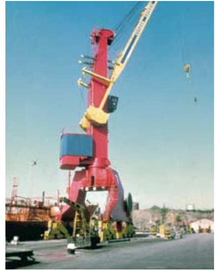
Crane with unbalanced boom, 15 ton/40 m.
